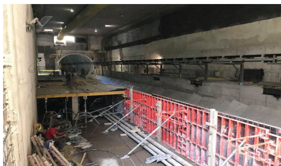
Construction of Metrostation III-11”Medical university Sofia”
