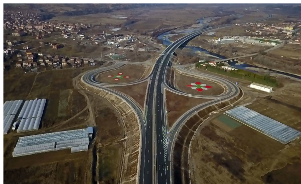
Struma Motorway, Road junction “Strumyani”
