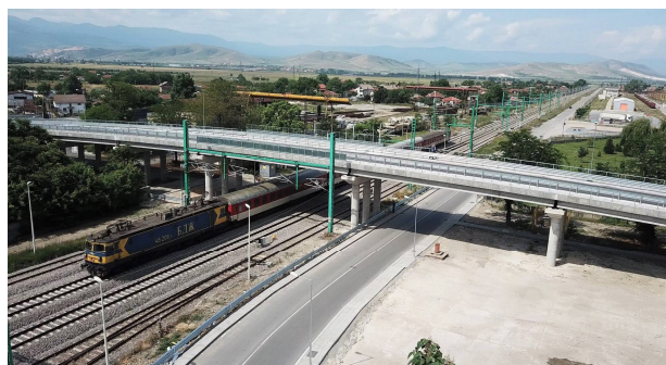
Road overpass in the area of town Stamboliyski
