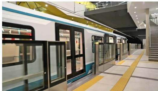
Automatic platform partition doors
