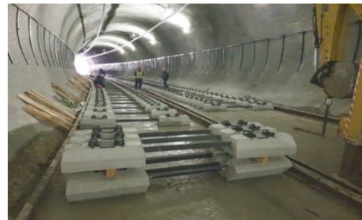
Laying of Metrolines
